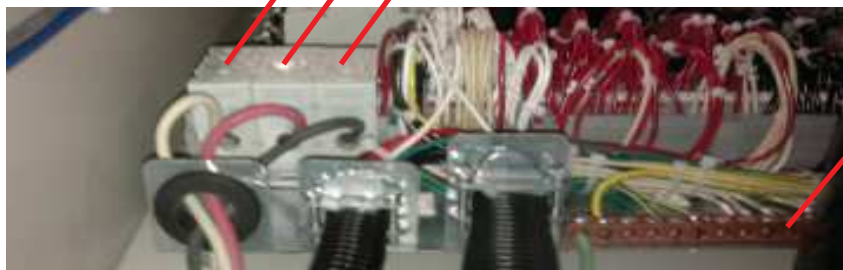
Figure 1. Power Distribution Block
